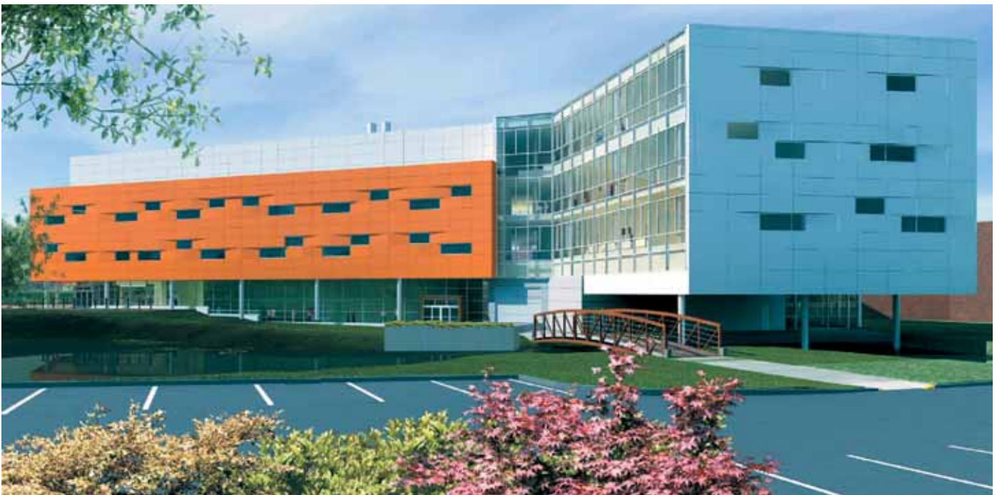
DCCC used energy modeling to aid in the design of the new STEM complex.
