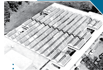
Flat-plate collectors were retrofitted onto the existing school rooftop.
